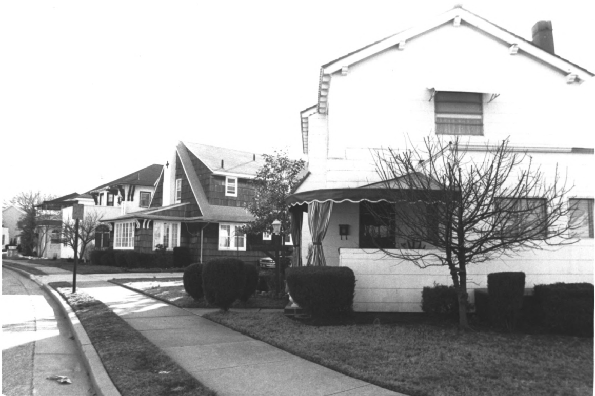
West side of East Drive North of Winchester Ave., Marvin Gardens Historic District, Margate, Atlantic County, N.J. # 28 of 34
