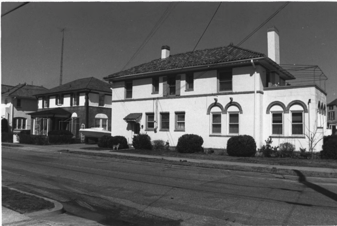
Brunswick Ave., from Ventura Ave., Martin Gardens Historic District, Margate, Atlantic County, N.J. #29 of 34
