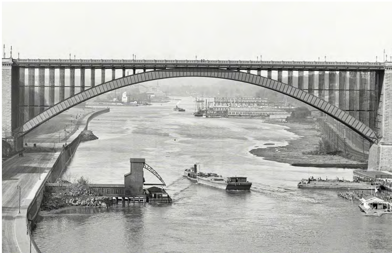
Figure 1. Northward view of Washington Bridge spanning Harlem River, c. 1905. The Morris Heights yard of Charles L. Seabury Co. and Gas Engine & Power Co., Consolidated is visible in the distance on the east side of the river. (Source: Shorpy.com, http://www.shorpy.com/node/19992 .)
