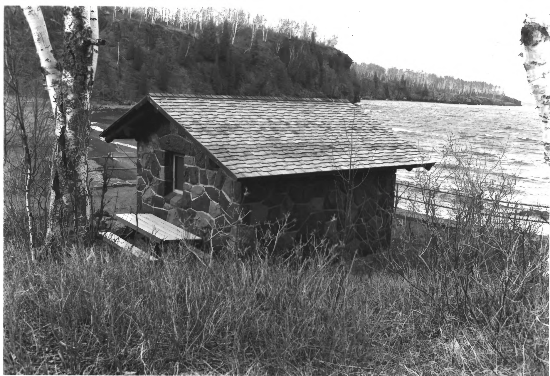
GOOSEBERRY FALLS STATE PARK LAKE CO. MN BLDG # 15 PHOTO I.D. 09765 # 2
