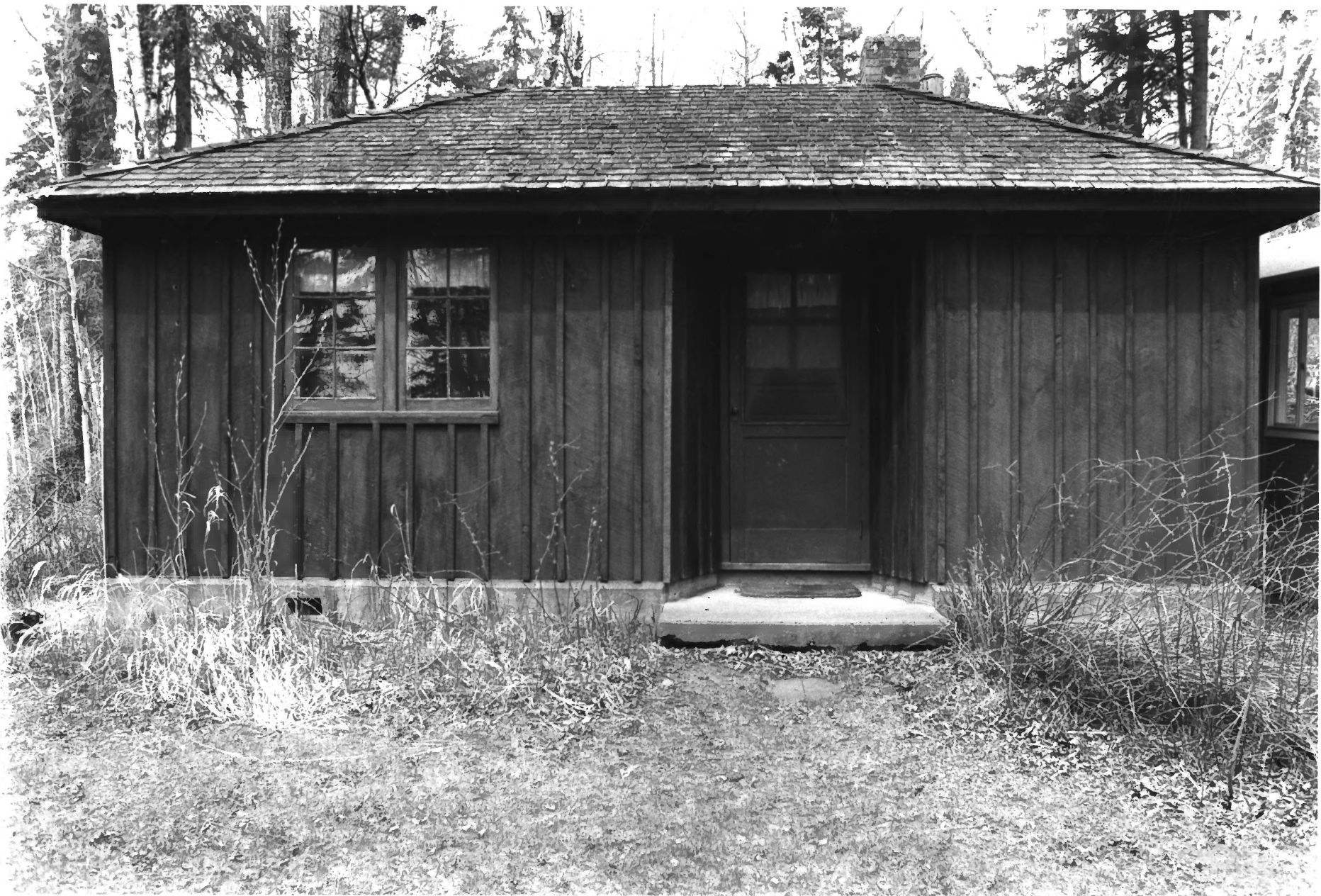
GOOSEBERRY FALLS STATE PARK LAKE CO., MN BLDG# 5 PHOTO I.D. 09767#7
