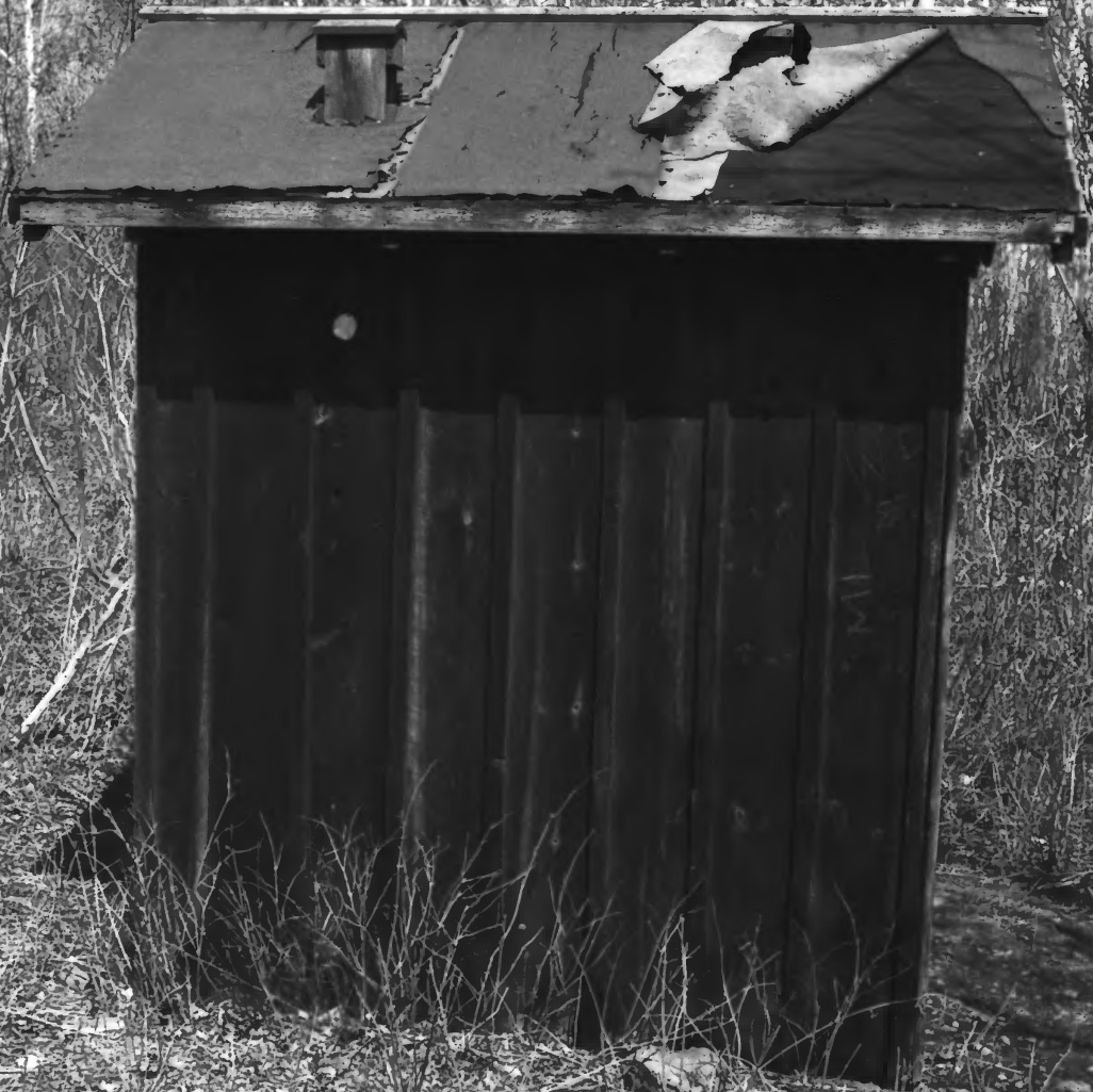
GOOSEBERRY FALLS STATE PARK LAKE CO. MN BLDG # 27 PHOTO I.D. 09768 # 24
