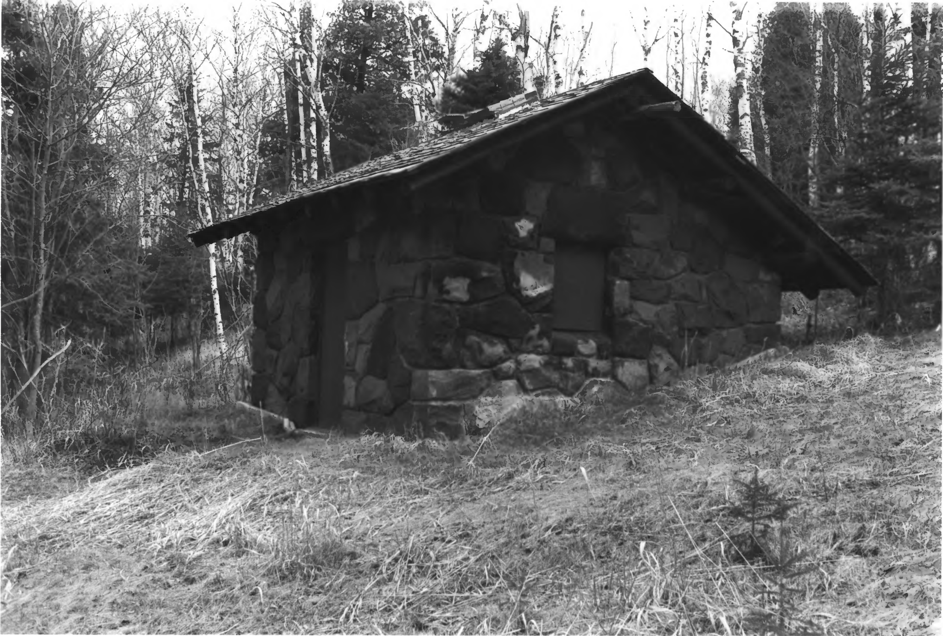
GOOSEBERRY FALLS STATE PARK LAKE CO., MN BLDG # 31 PHOTO I.D. 09767 # 23
