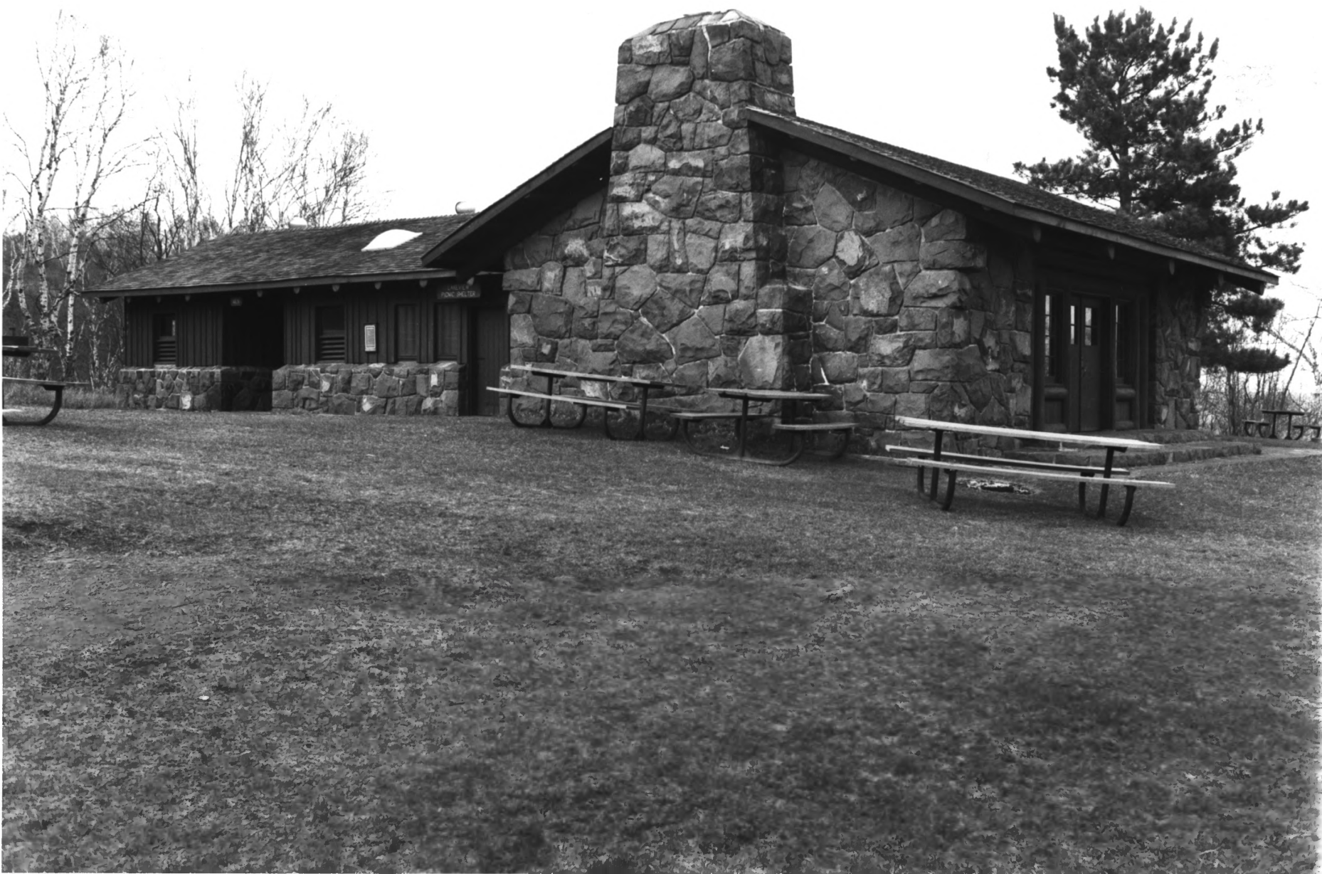
GOOSEBERRY FALLS STATE PARK LAKE CO., MN BLDG #13 PHOTO I.D. 09763 # 23
