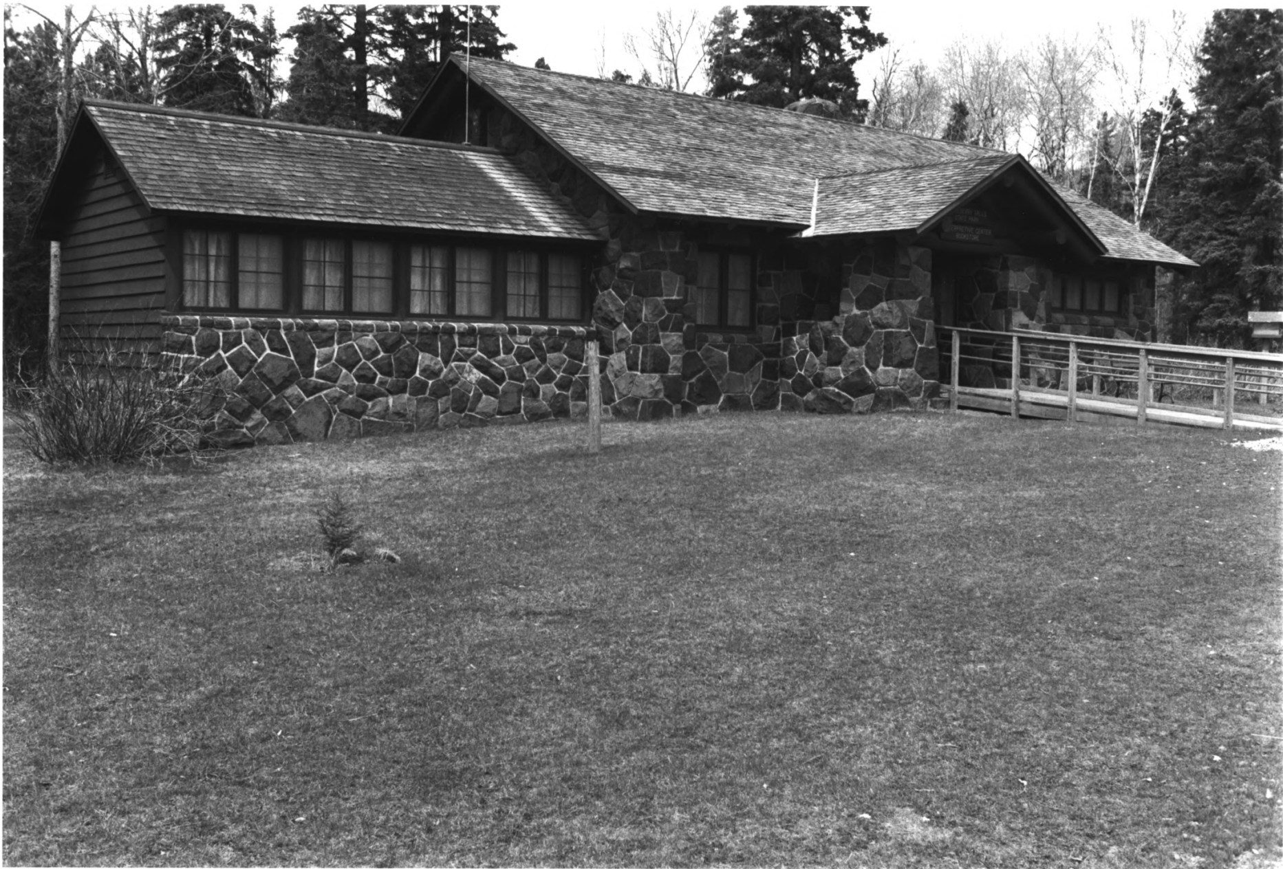
GOOSEBERRY FALLS STATE PARK LAKE CO. MN BLDG # 3 PHOTO I.D. 09767 # 13
