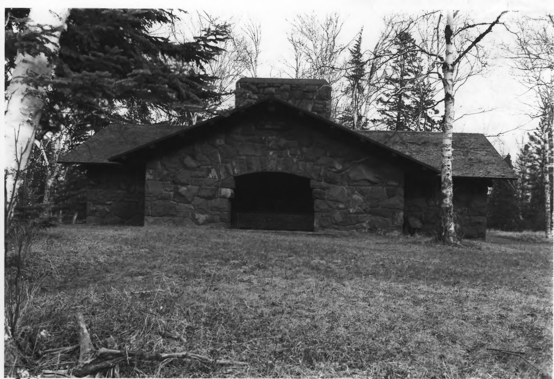
GOOSEBERRY FALLS STATE PARK LAKE CO., MN BLDG #12 PHOTO I.D. 09763 #18
