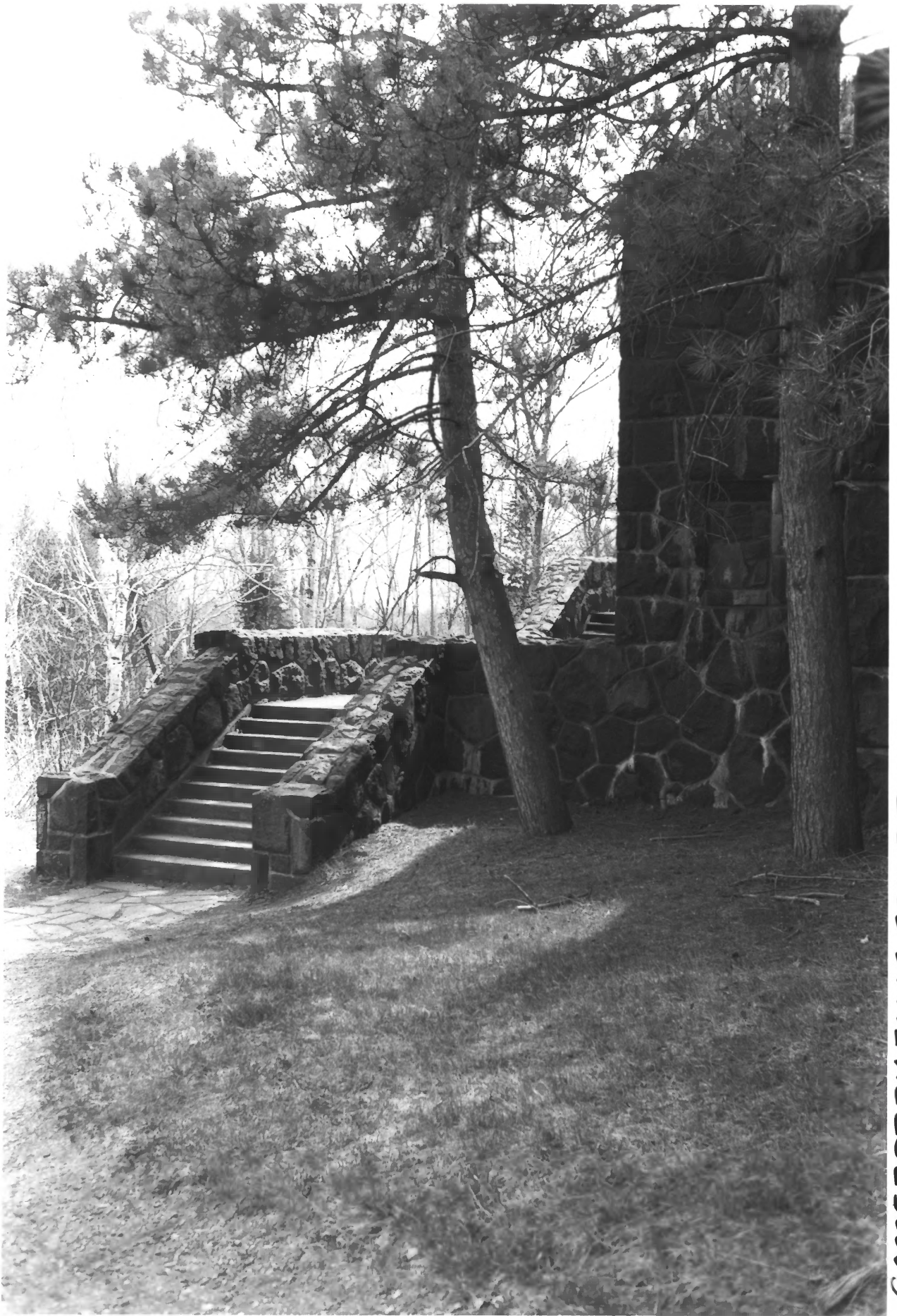
GOOSEBERRY FALLS STATE PARK - LAKE CO, MN STRUCTURE #1 PHOTO I.D. 09763 #7
