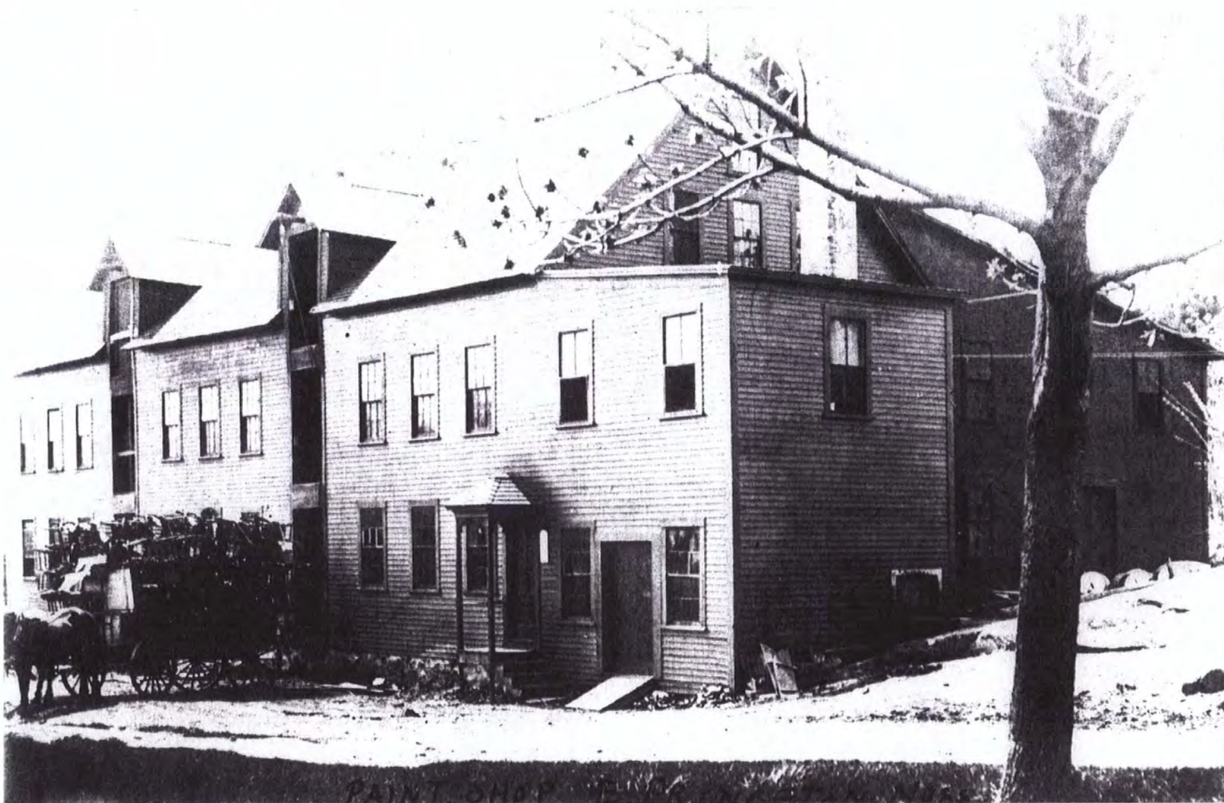
ILLUSTRATION # 9B Temple-Stuart Paint Shop, Gleason Road, c.1900 This view of the main façade was taken from Gleason Road, looking northeast. Finished chairs have just been loaded on a wagon from the warehouse loading doors to be taken to the Stuart Barn at 66 Main Street for Overnight storage before delivery to the railroad station for shipping the next day.
