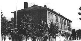
Cooper School, West Elevation C. 1930, Photo 216-03
