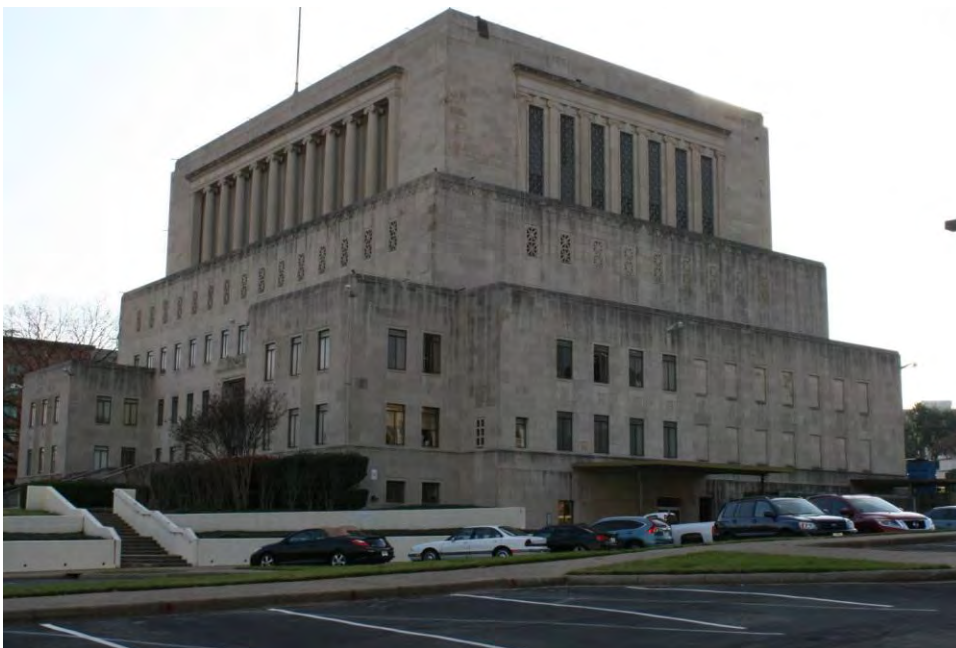
Photo 2: Façade and north elevation, January 8, 2016, looking southwest.
