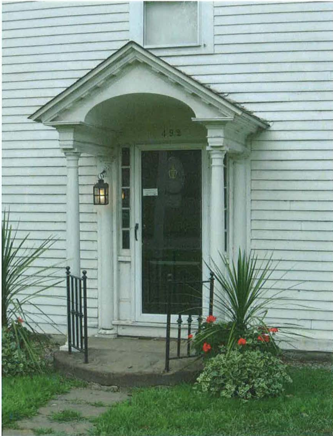
East (front) elevation of house from Main Street, showing entry details. Camera facing west. Photograph 8 of 27.
