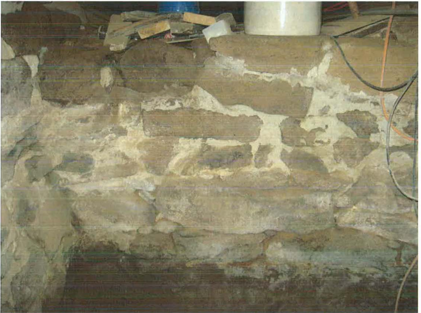
Interior of cellar, showing foundation detail. Camera facing north. Photograph 3 of 27.
