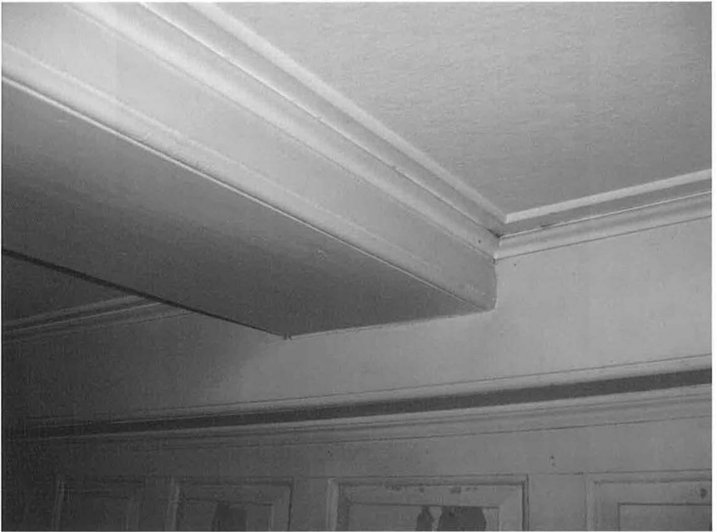
Interior of second-floor southeast bedchamber, showing wall paneling, and cased summer and girt details.
