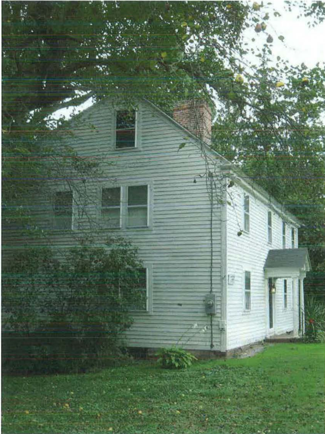
South (side) and east (front) elevations of house from Main Street, showing first- and second-story paired windows.
