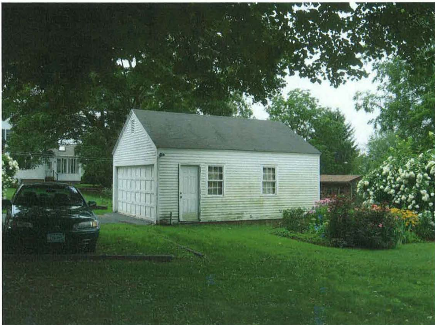
East (front) and north (side) elevations of Garage from rear of house, showing wall, door, and window details.
