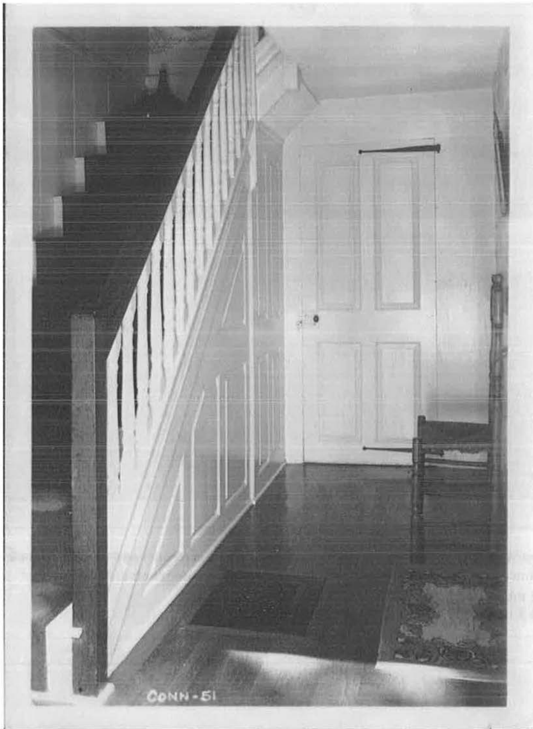
Works Progress Administration (WPA) photograph of the interior of the entry hall of 478 Main Street, showing stair, newel post, rail, baluster, paneling, and door details.
