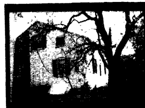
NE and NW elevs., looking SW
