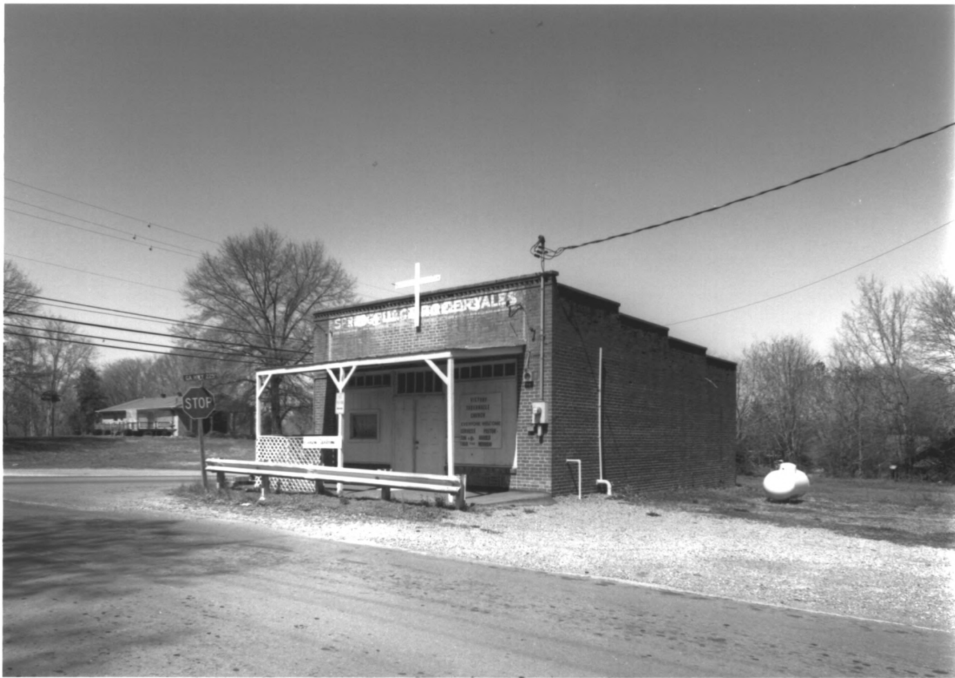
SPRING PLACE HISTORIC DISTRICT SPRING PLACE, MURRAY COUNTY, GEORGIA PHOTOGRAPH 10 OF 27
