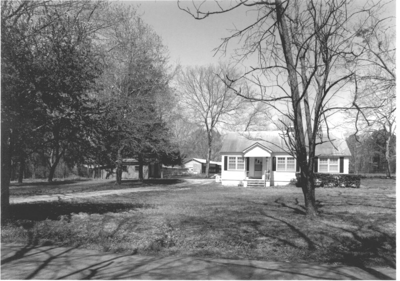
SPRING PLACE HISTORIC DISTRICT SPRING PLACE, MURRAY COUNTY, GEORGIA PHOTOGRAPH 16 OF 27
