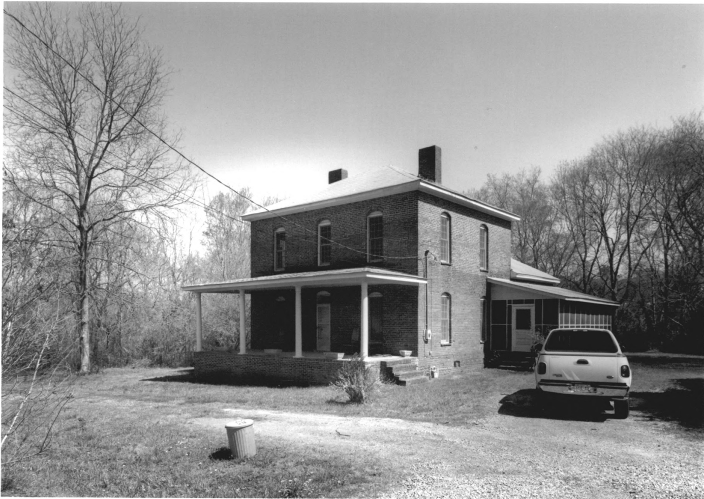
SPRING PLACE HISTORIC DISTRICT SPRING PLACE, MURRAY COUNTY, GEORGIA PHOTOGRAPH 11 OF 27
