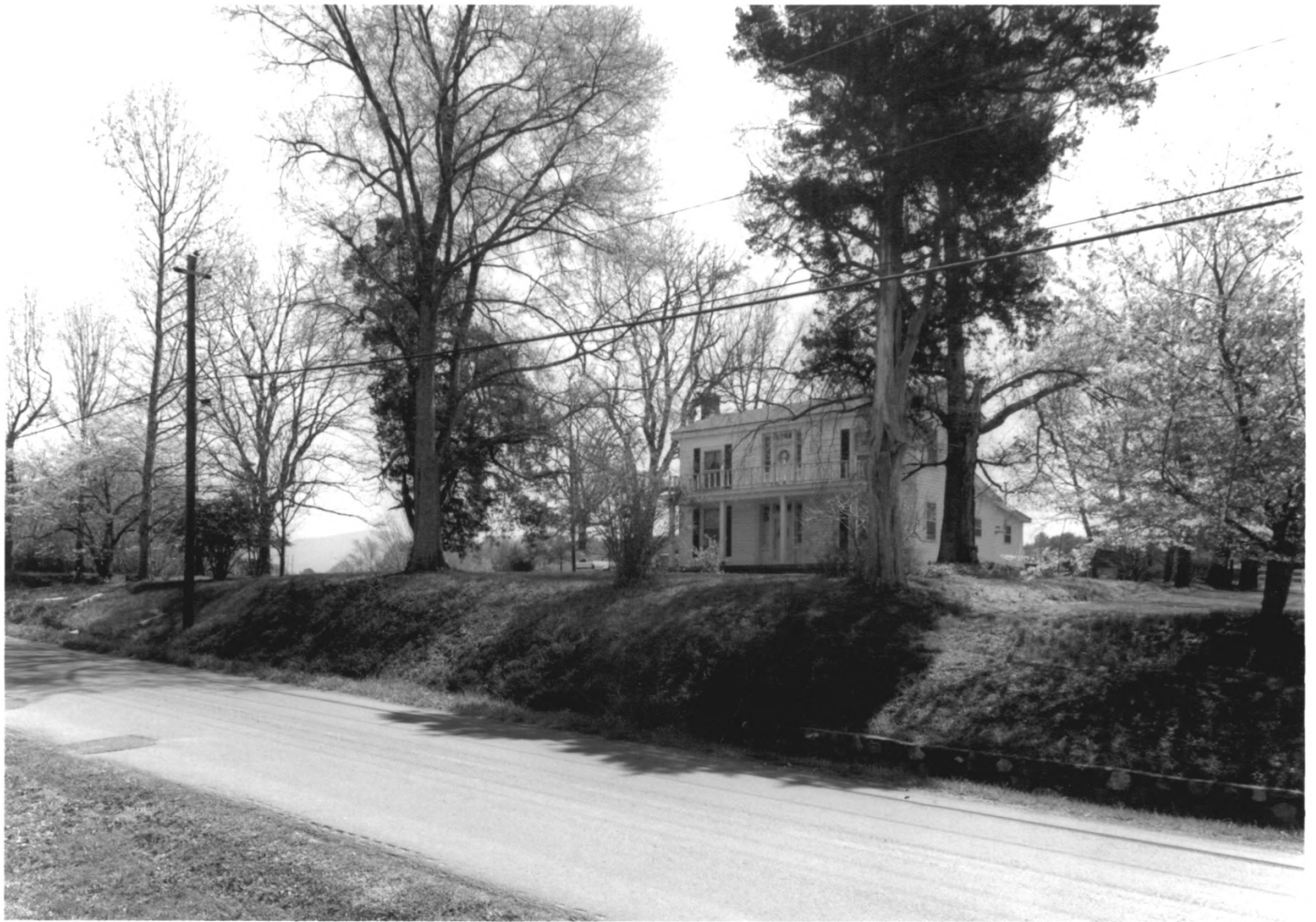
SPRING PLACE HISTORIC DISTRICT SPRING PLACE, MURRAY COUNTY, GEORGIA PHOTOGRAPH 19 OF 27
