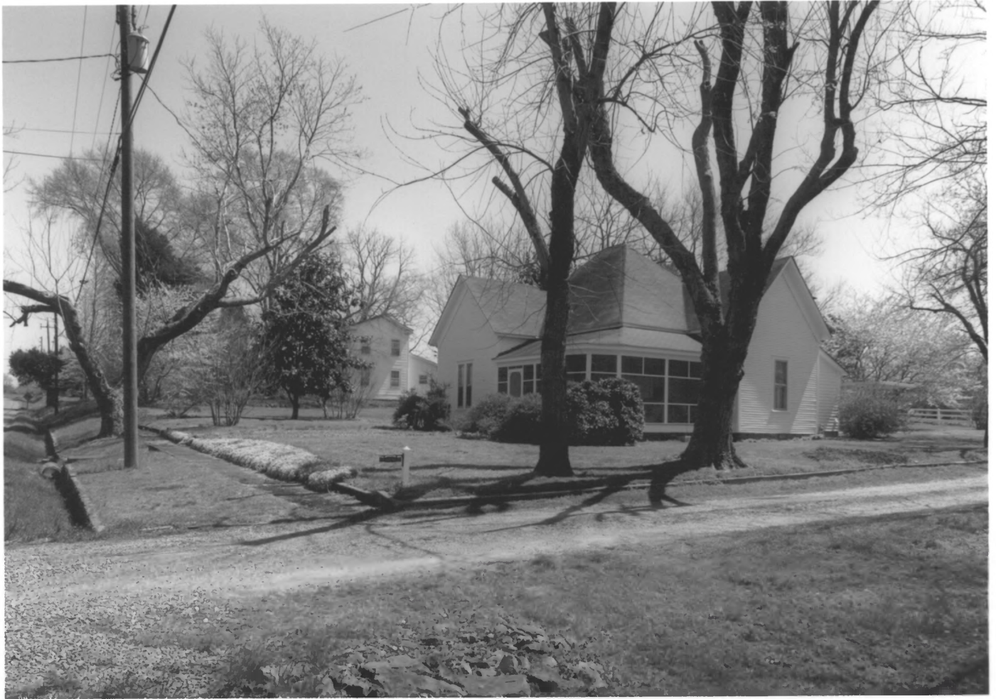
SPRING PLACE HISTORIC DISTRICT SPRING PLACE, MURRAY COUNTY, GEORGIA PHOTOGRAPH 18 OF 27
