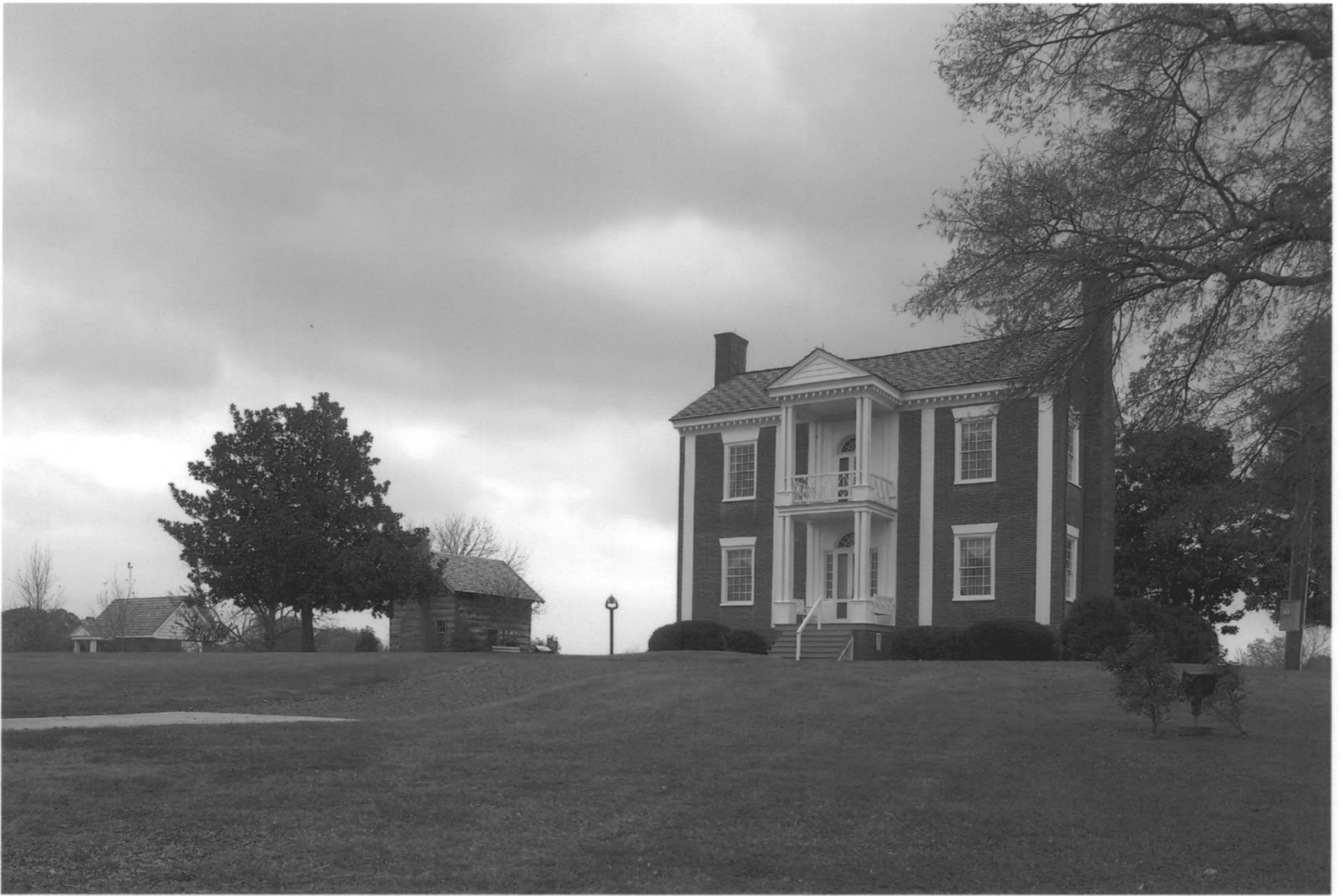
SPRING PLACE HISTORIC DISTRICT SPRING PLACE, MURRAY COUNTY, GEORGIA PHOTOGRAPH 24 OF 27
