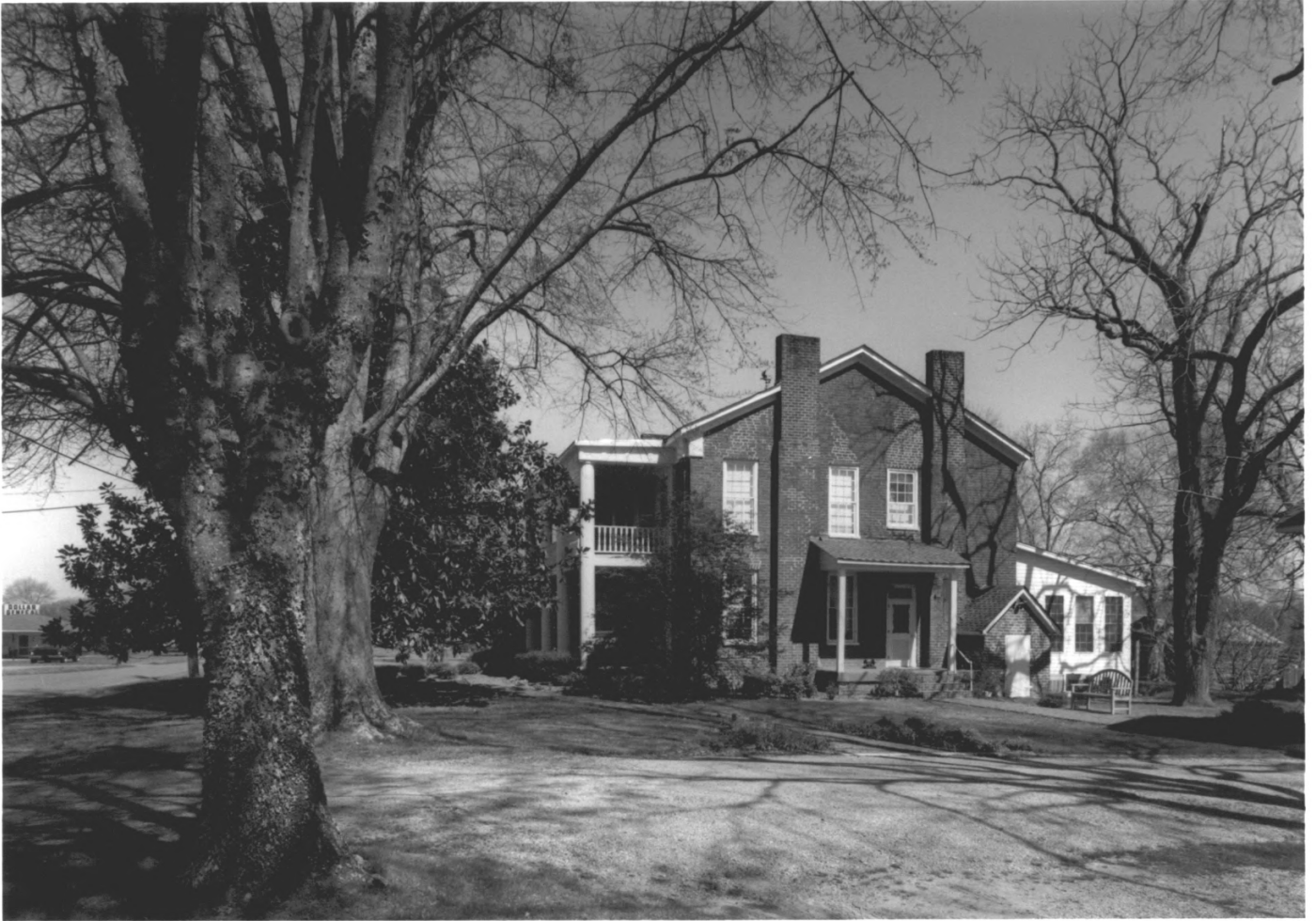
SPRING PLACE HISTORIC DISTRICT SPRING PLACE, MURRAY COUNTY, GEORGIA PHOTOGRAPH 4 OF 27
