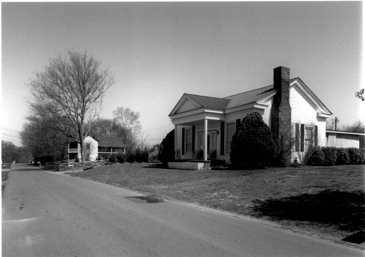
SPRING PLACE HISTORIC DISTRICT SPRING PLACE, MURRAY COUNTY, GEORGIA PHOTOGRAPH 8 OF 27
