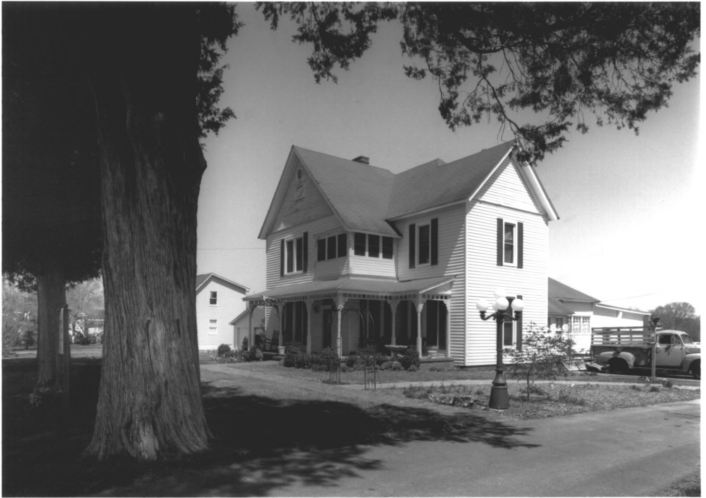
SPRING PLACE HISTORIC DISTRICT SPRING PLACE, MURRAY COUNTY, GEORGIA PHOTOGRAPH 6 OF 27
