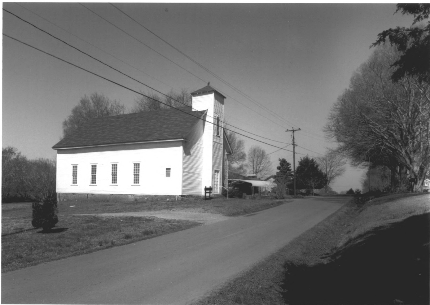
SPRING PLACE HISTORIC DISTRICT SPRING PLACE, MURRAY COUNTY, GEORGIA PHOTOGRAPH 1 OF 27
