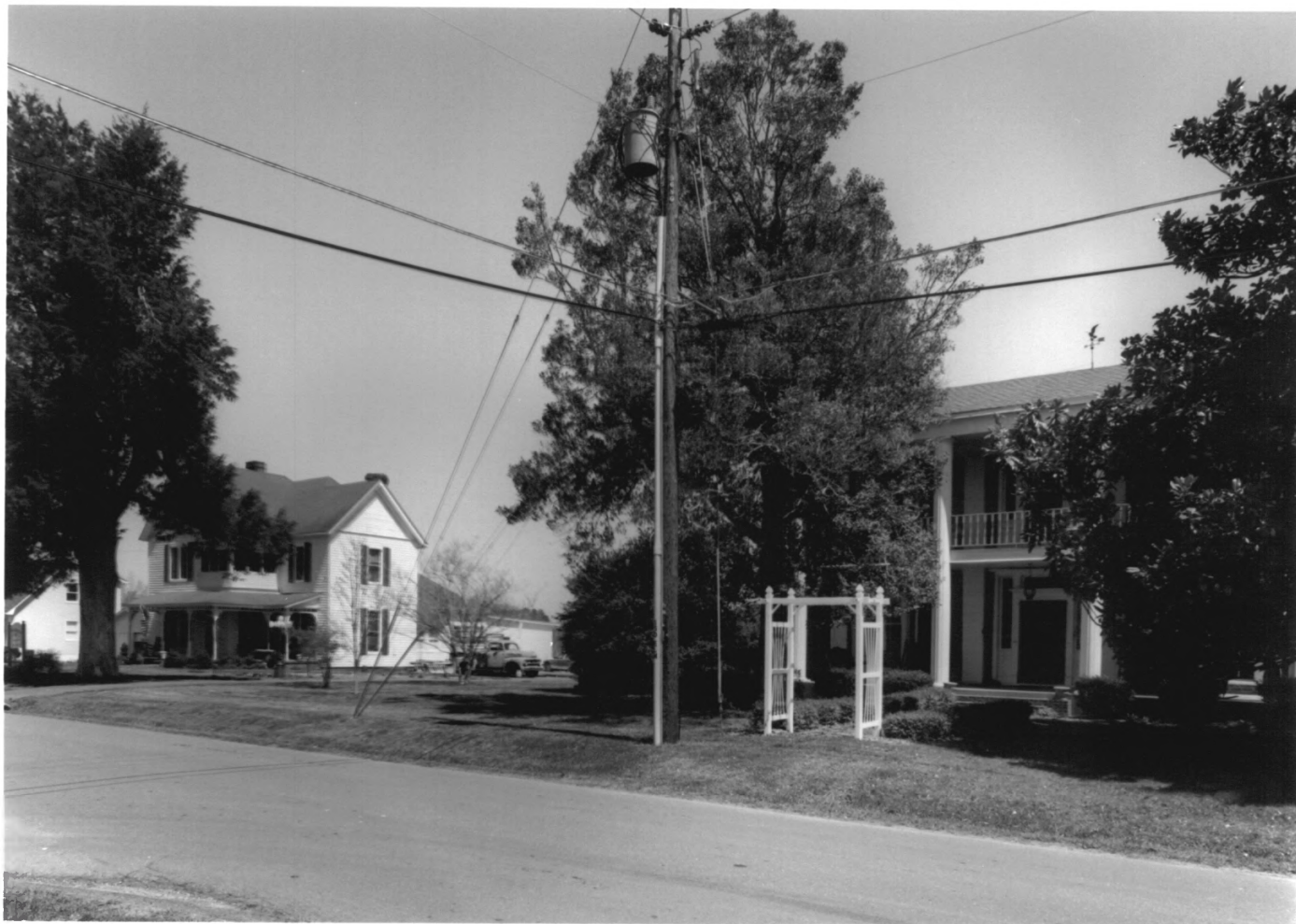
SPRING PLACE HISTORIC DISTRICT SPRING PLACE, MURRAY COUNTY, GEORGIA PHOTOGRAPH 3 OF 27
