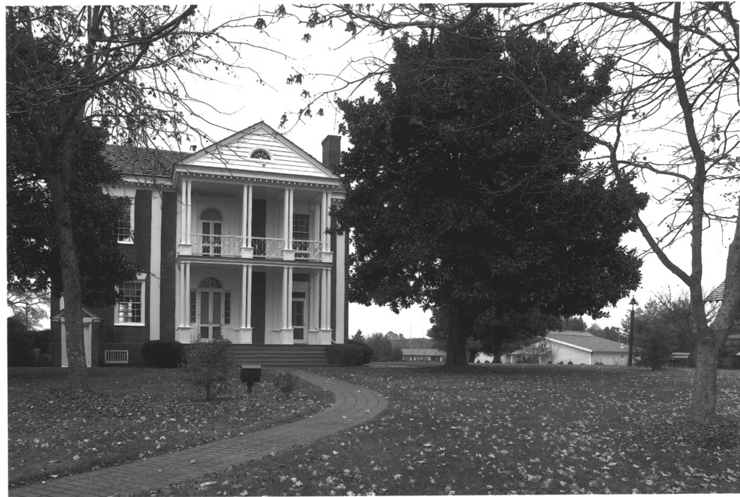
SPRING PLACE HISTORIC DISTRICT SPRING PLACE, MURRAY COUNTY, GEORGIA PHOTOGRAPH 27 OF 27
