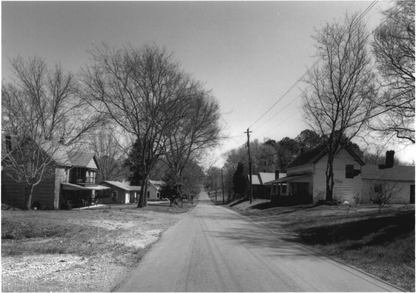
SPRING PLACE HISTORIC DISTRICT SPRING PLACE, MURRAY COUNTY, GEORGIA PHOTOGRAPH 12 OF 27
