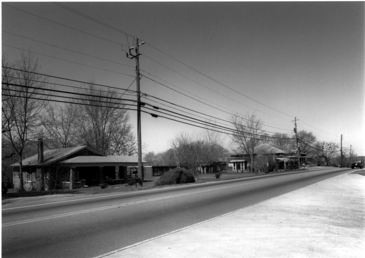
SPRING PLACE HISTORIC DISTRICT SPRING PLACE, MURRAY COUNTY, GEORGIA PHOTOGRAPH 9 OF 27
