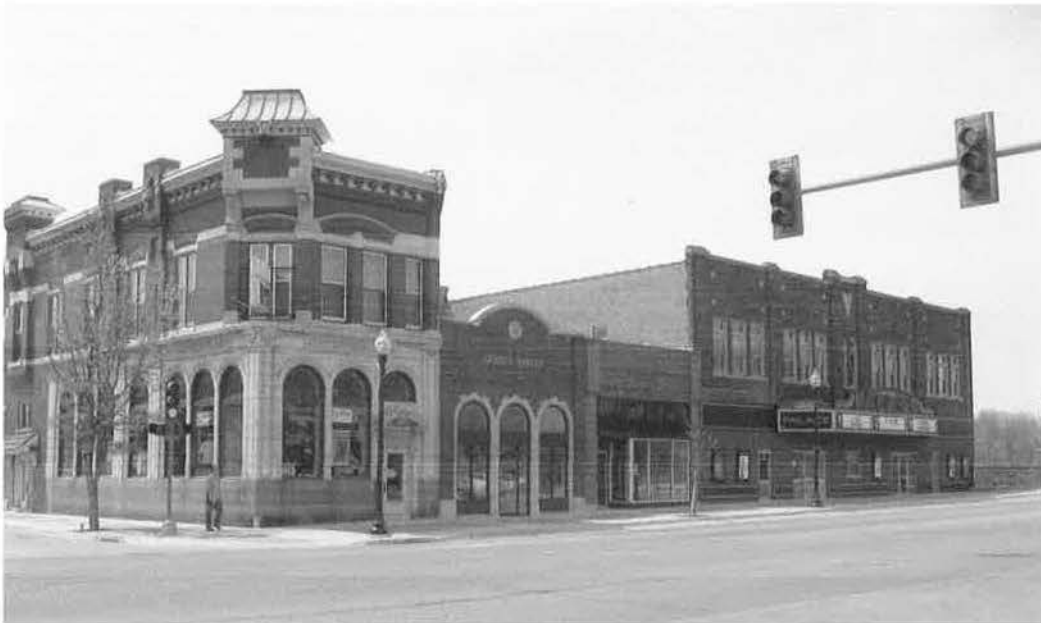
Figure 2 - L to R: 98, 96, 94, 92-88 East Bremer Avenue (92 is a current postal address for a small office within the larger theater building)
