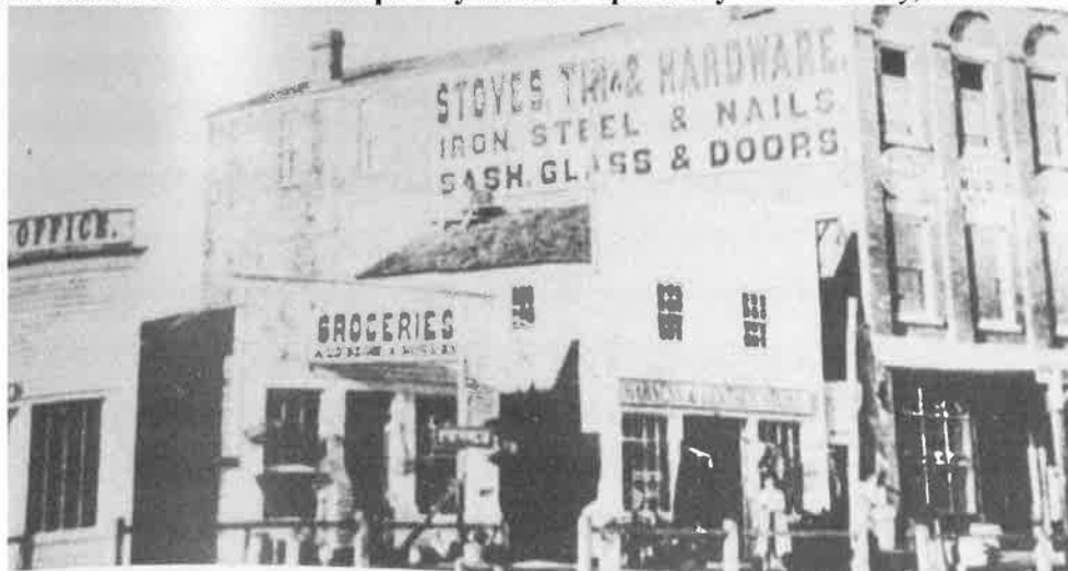
Figure 28 Small wooden false-front store buildings like those seen here on the south side of the 100 block of East Bremer Avenue are typical of the first generation commercial structures built in new Iowa towns. This photo is undated but was taken between 1865 and 1869, based on the construction dates for the buildings that replaced them. Eventually, these wood-frame stores gave way to larger and more fireproof buildings in growing, economically robust towns. The tall building on the right is the extant S.H. Curtis Hardware store (began in 1855 at 116 East Bremer Avenue). Waverly, Rich in Iowa Heritage [1996], 59.
