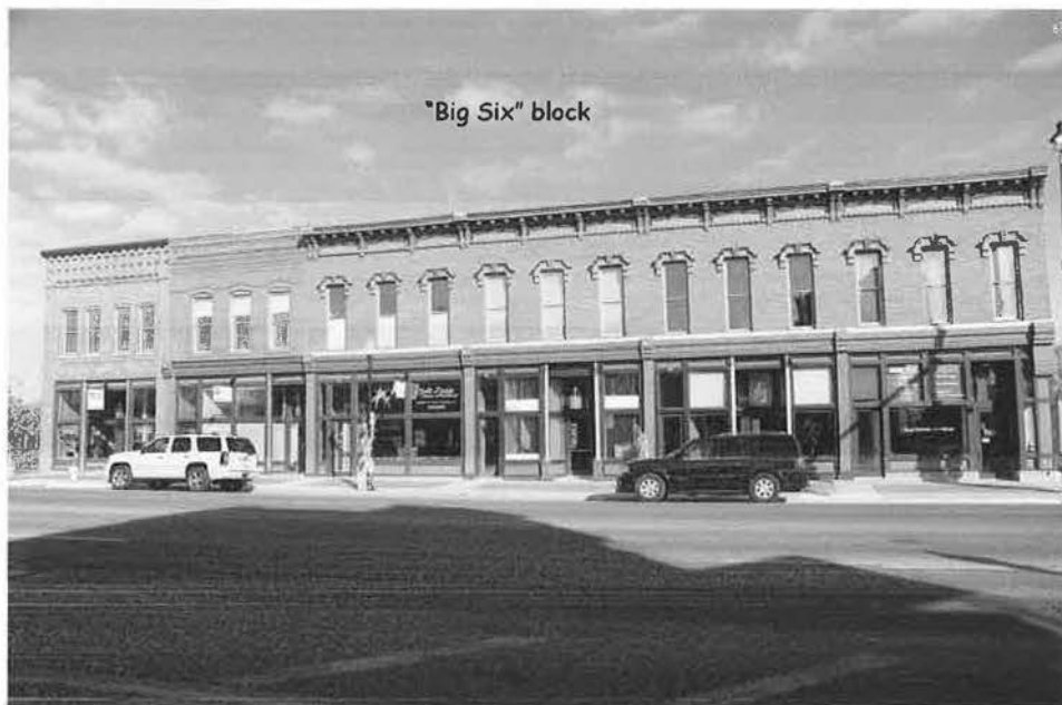
Figure 1 - L to R: 89, 91, 93, 95, 97, and 99 East Bremer Avenue
