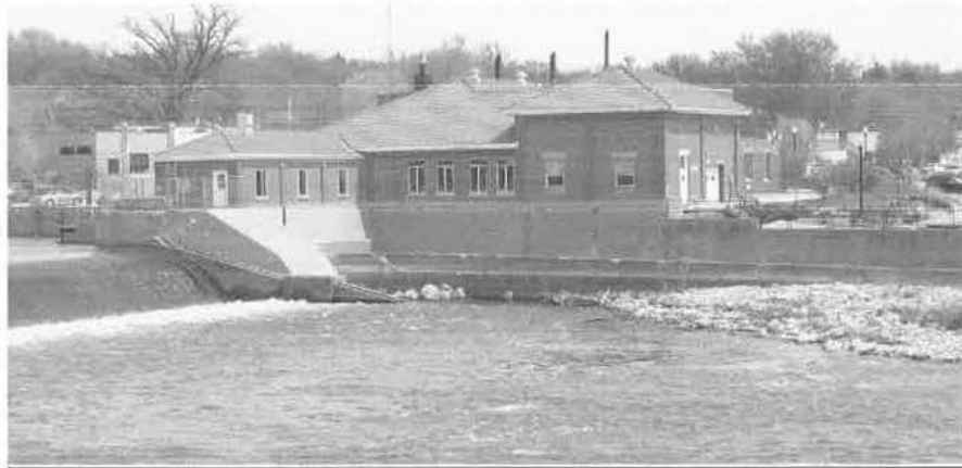
Figure 4 – Waverly Municipal Hydroelectric Powerhouse
