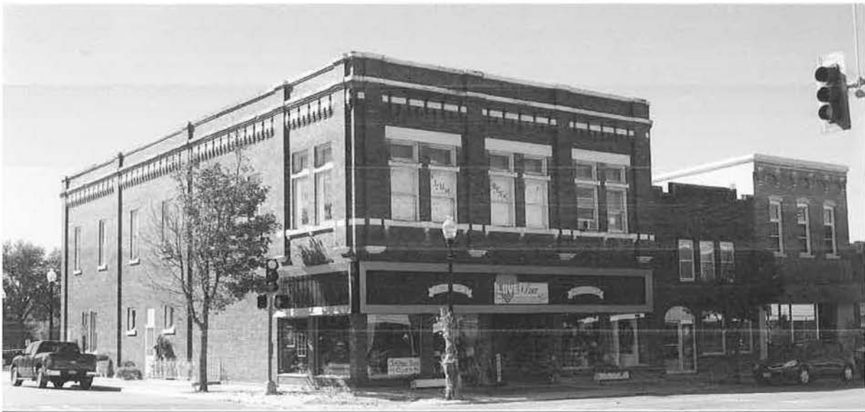
Figure 12 – L – R: 220, 218, 216 East Bremer Avenue
