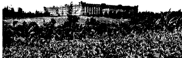
Partial view of northern and western façade. c. 1939
