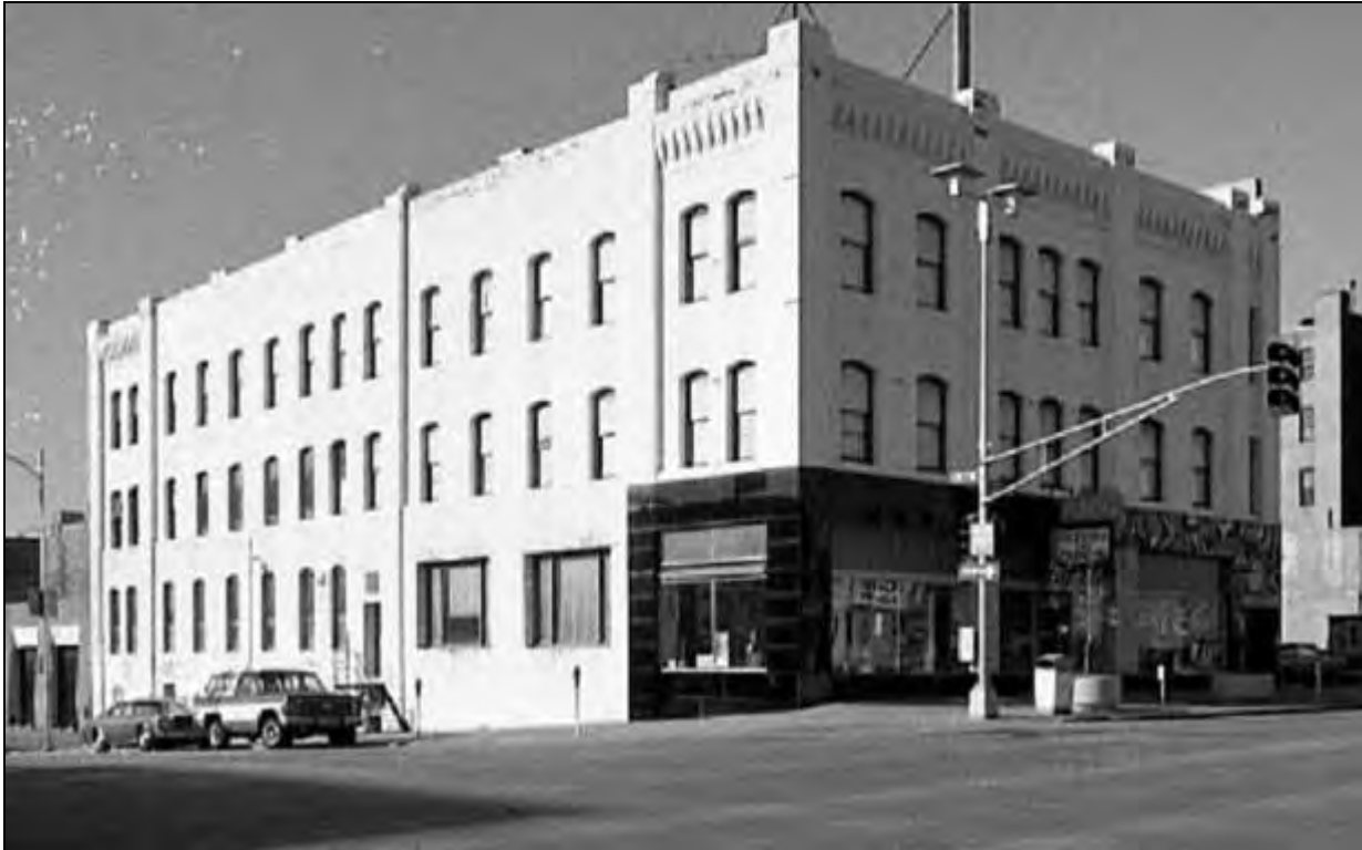
Figure 16: The SOTA building occupied by “Bobbitt Moulding and Frame Company” circa 1980. Note the glossy dark tiles around the ground floor entrance/display windows, and the lack of light wells/railings on the side (east) elevation.
