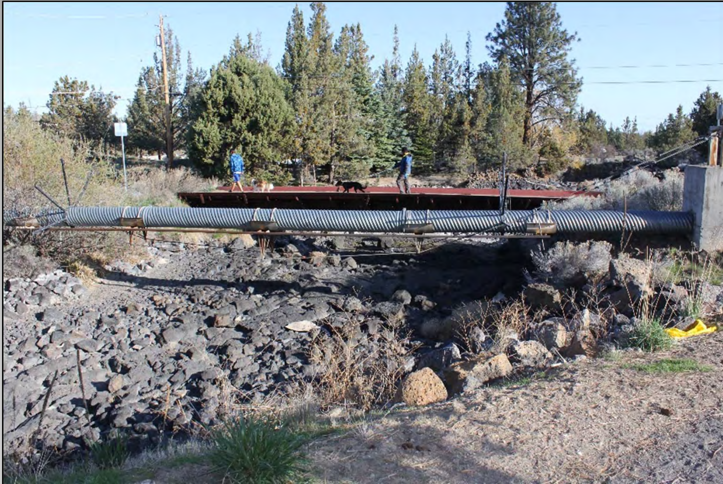
Yeoman Road Pedestrian Bridge
