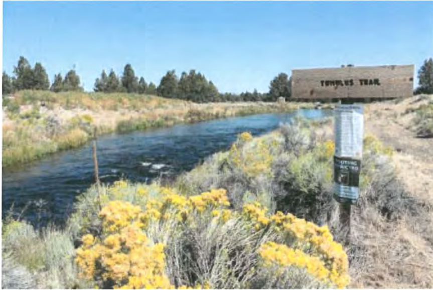
The “I” Lateral in Alfalfa, looking southeast, August 2016.
