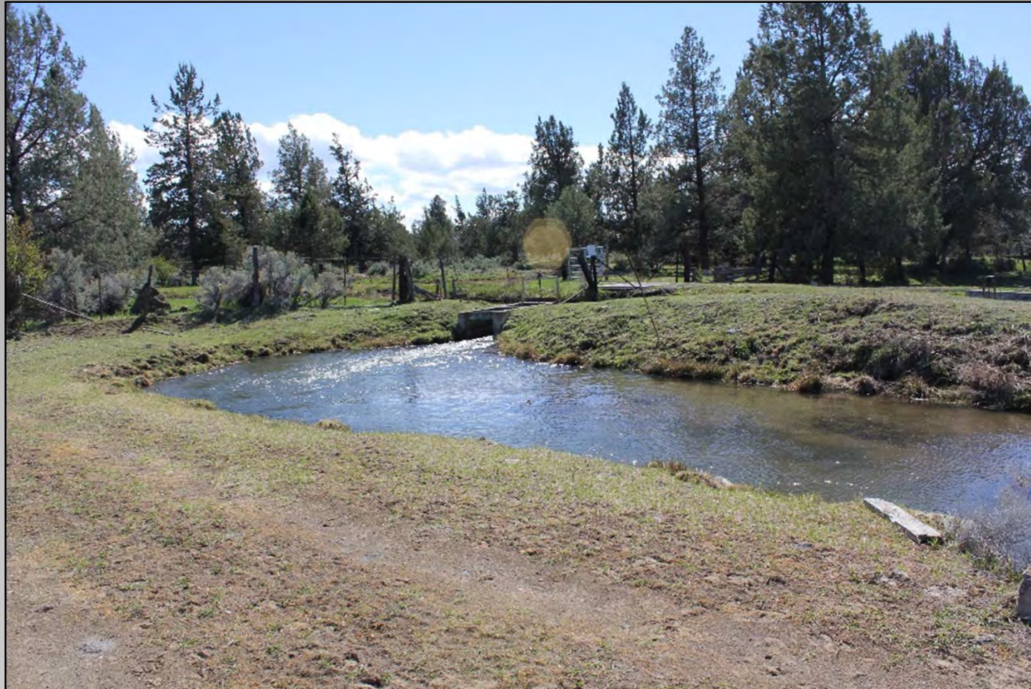
End of the Pilot Butte Canal near Smith Rock State Park
