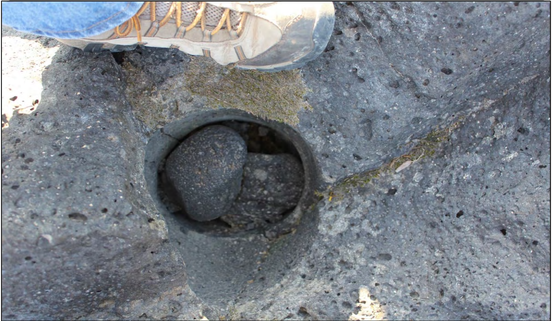
A hole drilled for explosives from 1904 in the canal.
