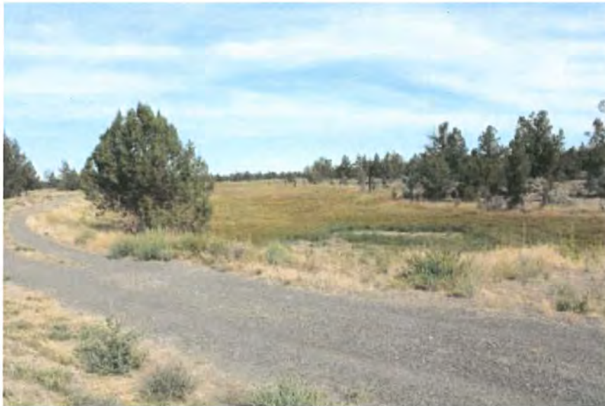
Piped “I” Lateral near Zell Pond. The road is on top of the pipe. Looking northwest away from Zell Pond.
