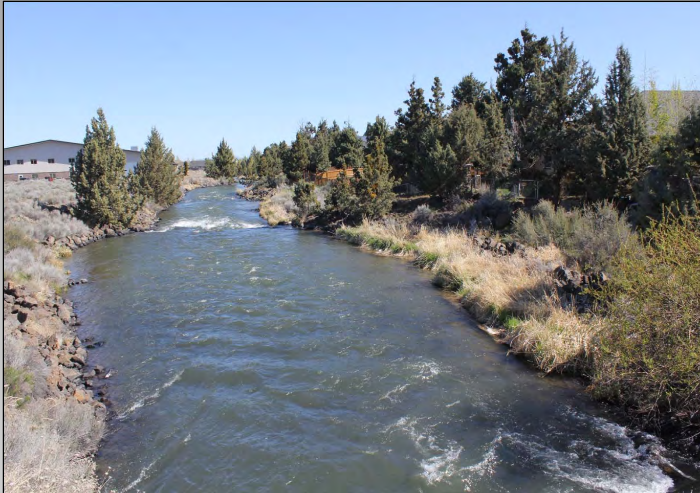
The 1904 Pilot Butte Canal at Brinson Blvd. Bridge. No abutments, two cuts on sides, rocky bed, scattered riprap, silt.
