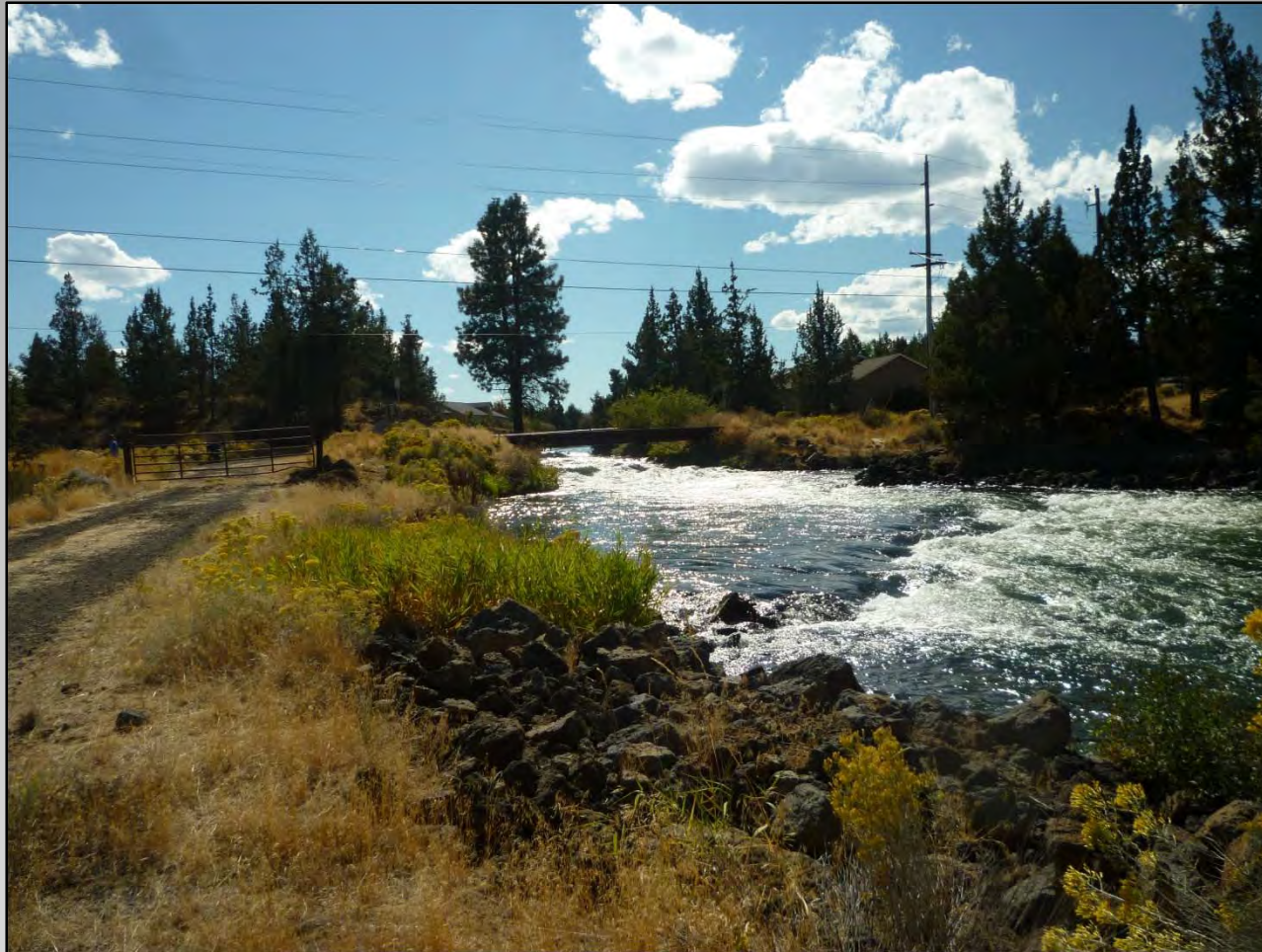
Southern edge of the Pilot Butte Canal Historic District. Listed on the National Register of Historic Places 2016
