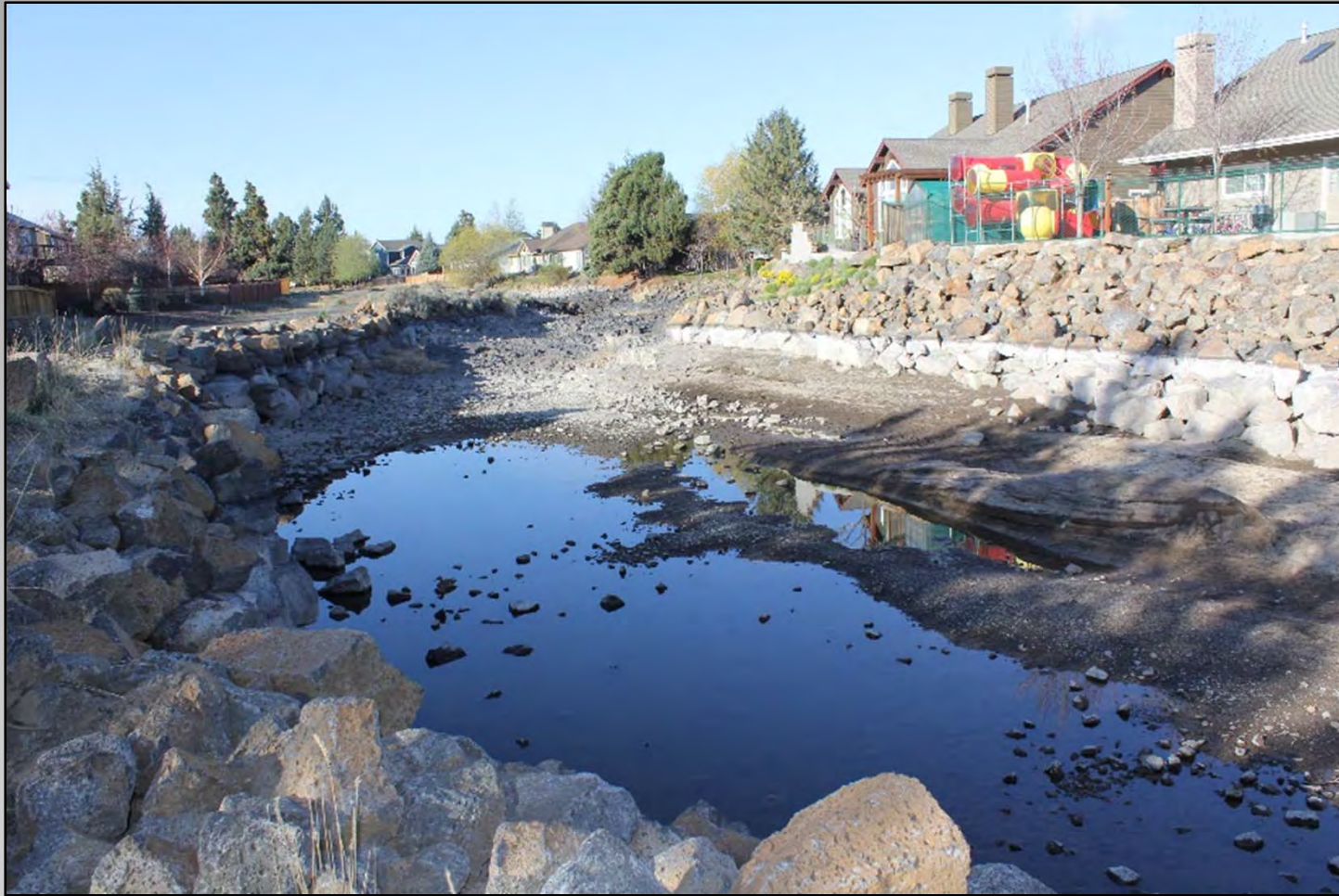
New retaining walls run into sides of canal.
