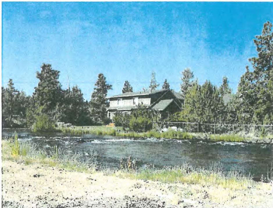
Overview of residential properties encroaching on COID canal easement – both house and fenced yard are within easement.
