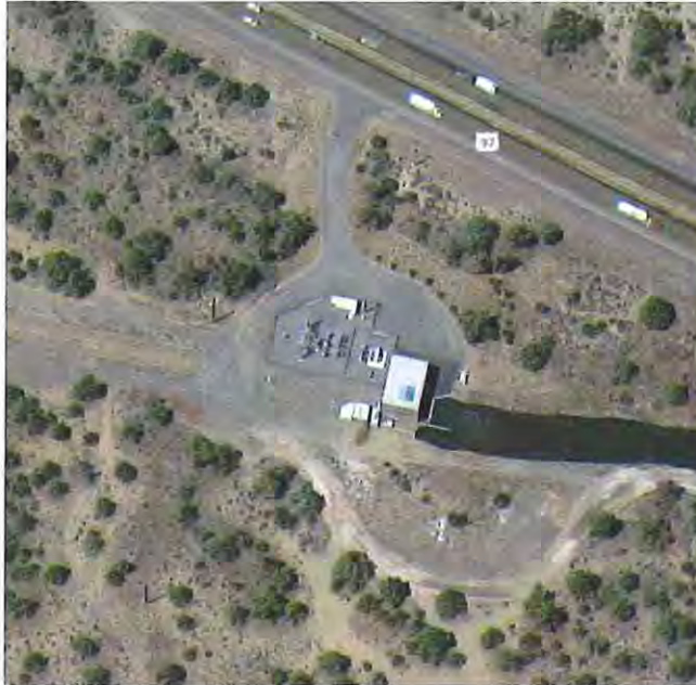
COID Hydropower Generator on the Pilot Butte Canal Source: Google Maps
