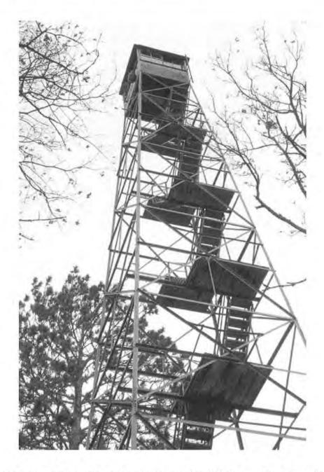
Figure F11. The Sandy Lake Tower is a stair tower with steps that climb the tower from side to side. The 100' tower was built in 1933 by either the WPA or SERA for the Minnesota Forestry Division. It is a rare example of a tower built by a New Deal agency other than the CCC. The tower is located at Sandy Lake Ranger Station, an early state ranger station. It is one of few towers remaining in the state that was fabricated by the Pittsburgh-Des Moines Company. 2014 photo by Gemini Research.
