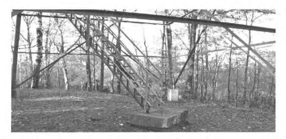
Figure F16. The stairs and their concrete footing at the Ben Draper Tower. The tower was erected by the CCC for the Minnesota Forestry Division in Land O'Lakes State Forest, which was established in 1933. It is a 100' tower fabricated by Aermotor. The 42" by 48" footing is signed and dated by the CCC. The tower is 24' square at the base and its largest members are 5" steel angles. 2014 photo by Gemini Research.
