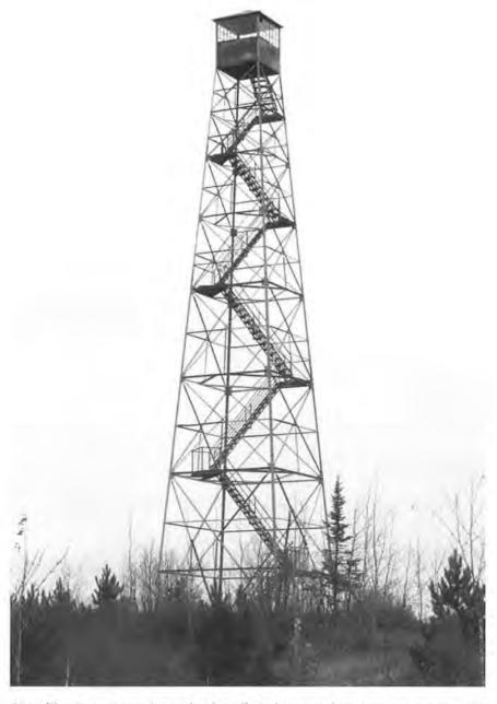
Figure F12. The Vermilion Dam Tower has stairs that climb the tower from corner to corner. There are both rectangular and triangular landings. It is an 86' tower manufactured by McClintic-Marshall. The Vermilion Dam Tower was built in 1934 by the CCC for the Minnesota Forestry Division. It stands in Kabetogama State Forest, created in 1931. Note that the hilltop has been cut or burned and is regrowing. 2014 photo by Gemini Research.
