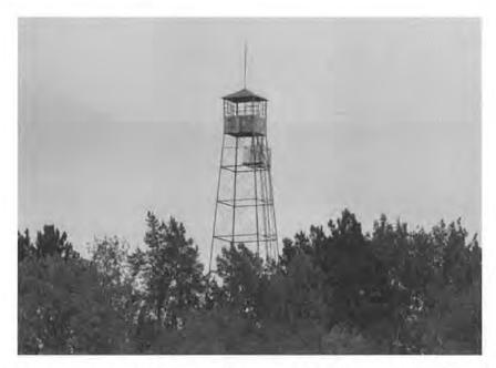
Figure F13. The upper portion of the Farley Hill Tower, erected in 1935. Farley Hill is a 100' ladder tower manufactured by Aermotor. It has an uncommon window glazing pattern. The early rooftop antenna provided two-way radio communication between the tower and the ranger station. 2014 photo by Gemini Research.
