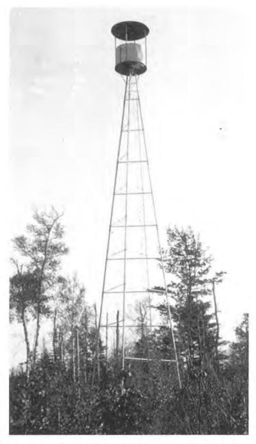
Figure F3. Some of Minnesota's earliest steel towers, like the unidentified example shown here, had three rather than four legs. The first cabs on steel towers were cylindrical, enclosing the open crow's nest. No examples of three-legged towers or towers with open platforms or cylindrical cabs have survived. Minnesota Historical Society collection.
