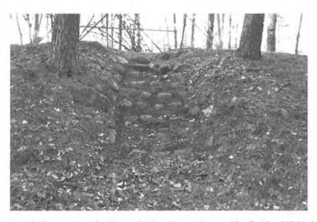
Figure F21. Rare CCC-built stone steps leading to the Ben Draper Tower. The flanking hillside is riprapped with stones. 2014 photo by Gemini Research.
