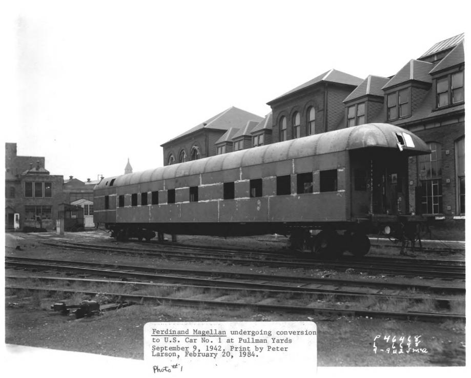
U.S. Presidential Pullman During this part of the "Ferdinand Magellan". construction the F.M. is Installation of 5/8 inch supported by "shop" armor plating, Sept. 1942. Photo taken Sept. 9,1942. trucks for movement within the Pullman yards. Printed Feb. 20, 1984.
