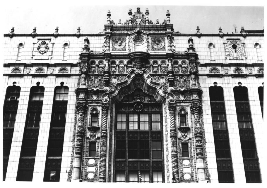
PHOTO 3 Detail of facade, showing "Frontispiece," or central bay stories two through six. Note pairs of elaborate columns on either side, decorative treatment of small windows between columns and decorative metal window spandrels in center and side bays.
